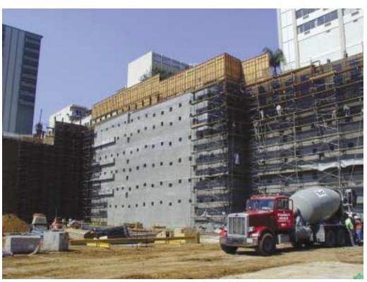
Partially completed Hollywood & Highland project in Hollywood, Calif. This project required over 13,000 yd<sup>3</sup> of 25-in.-thick shotcrete walls. A section of sawcut preconstruction panel for the project showed complete encasement of the reinforcing steel, even with lap-spliced #11 bars
